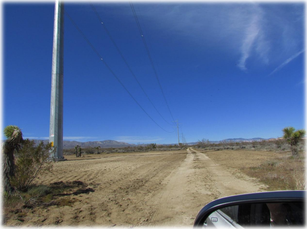
Photo 2: Baugh property easement showing mid-day shading, March 2, 2011
