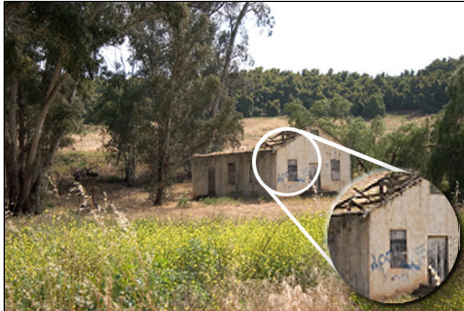
VANDALS HAVE DEFACED THIS HISTORIC HOUSE. PHOTO: SAVE OUR HERITAGE ORGANISATION
